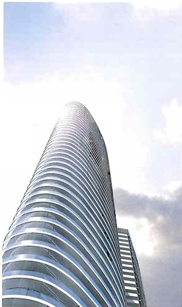
BLOCK 3 HOWARD 3B BUILDING
