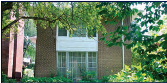
The proposal calls for the demolition of this house at 29 Sherbourne St. N.
