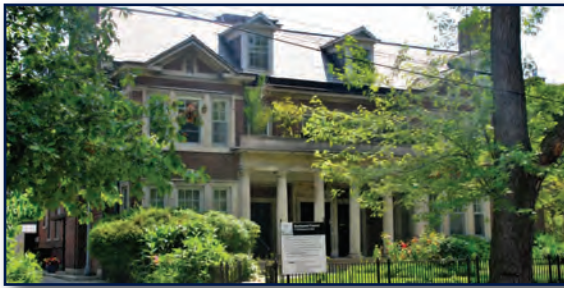
An addition is proposed for the rear of this building as part of the redevelopment of 21-35 Sherbourne St. N.
