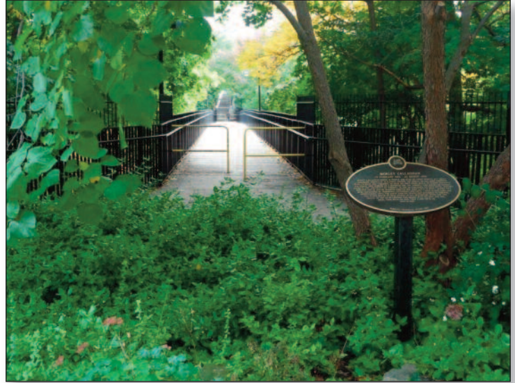
Glen Road Bridge in South Rosedale
